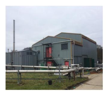
Demolition of the buildings were of a sensitive nature as for all the G/Waste generated from the works was stock piled and put through a shredder to go offsite as an energy from waste, and all scrap generated was processed onsite and went directly to smelter. All waste transfer notes corresponded with waste stream controlled by Ron Hull Demolition Ltd, all brick/concrete was transported to the laydown area for processing and crushed to a 6f2 material to be utilised onsite by the client.
